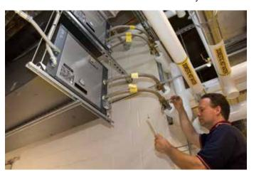
The original bid design of the mechanical system had a single outdoor unit for each building, to be fed by 460 volt, three-phase power. It was later determined that there was only 240 volt, single-phase power to the building. This changed the design substantially and meant that we had to go with multiple units of a smaller capacity. Due to the lack of three-phase power, the engineer's design called for two heat pumps in series with one another, with a third as stand-by.
