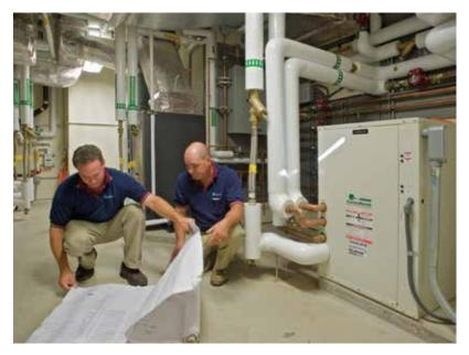
In the event of failure, or if outdoor temperatures falls below the 8°F system design temp, the building's water-to-air system kicks in as a source for back-up heat. The same units act as the building's AC system during the summer months.
