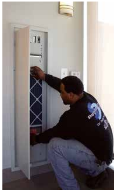
A technician installs a ClimateMaster vertical stack unit in the Alta
