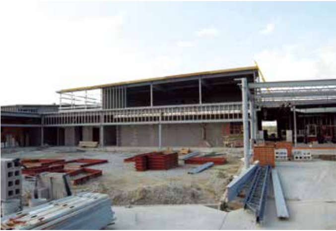
Construction in progress on the school grounds.
