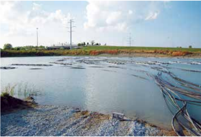
Loop Coils prepared for submersion into the pond.
