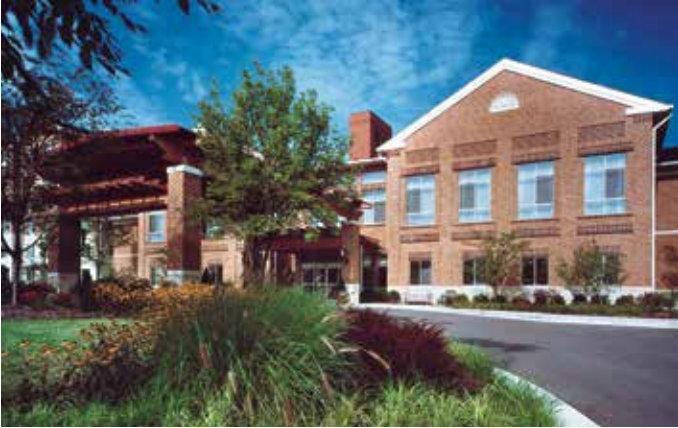
Riderwood Village began construction in 1998. This Erickson property is located in Silver Springs, Maryland, just minutes from Washington, D.C.
