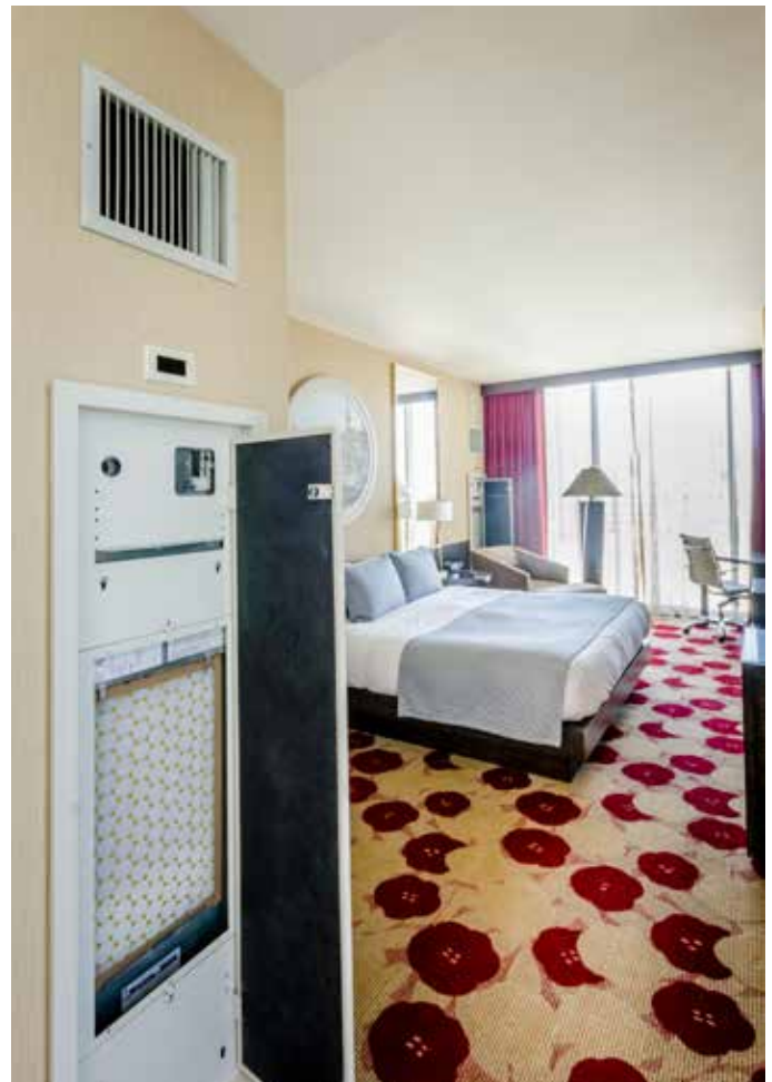
The VHS units make replacing air filters quick and easy.
