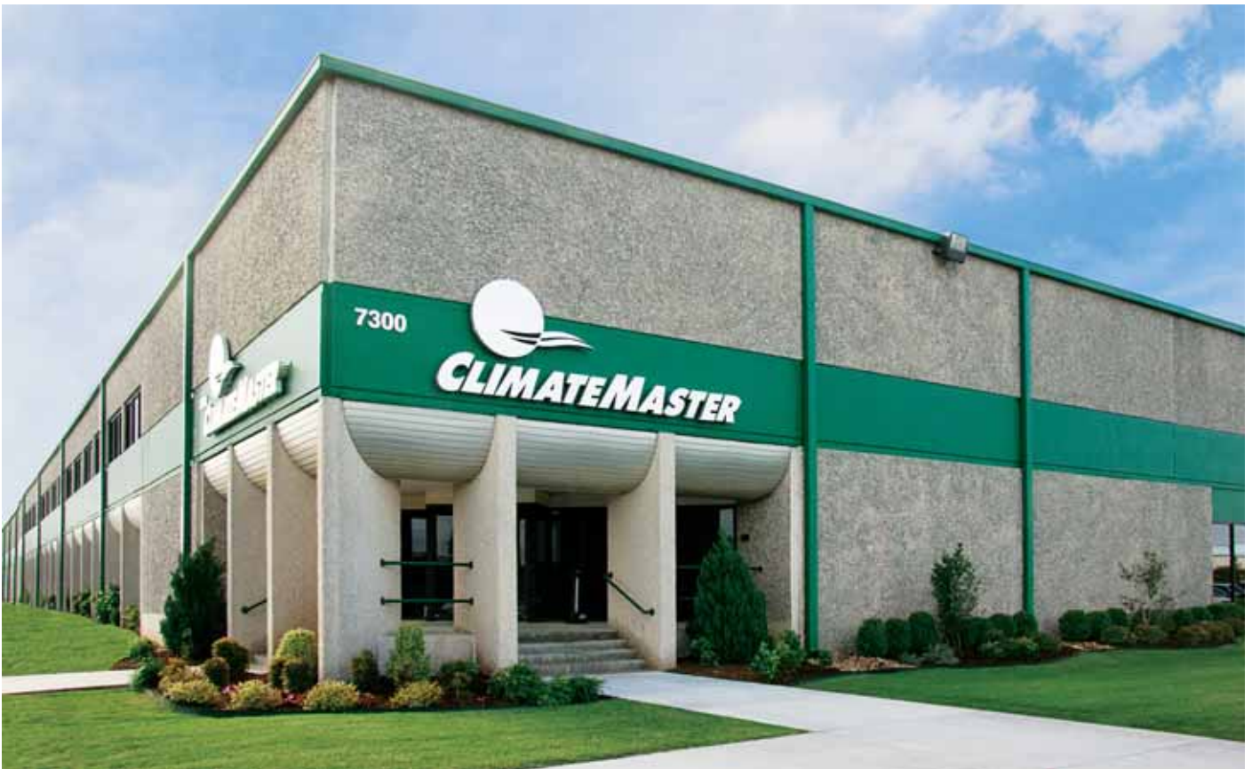
ClimateMaster's manufacturing facility in Oklahoma City, Oklahoma, U.S.A.
