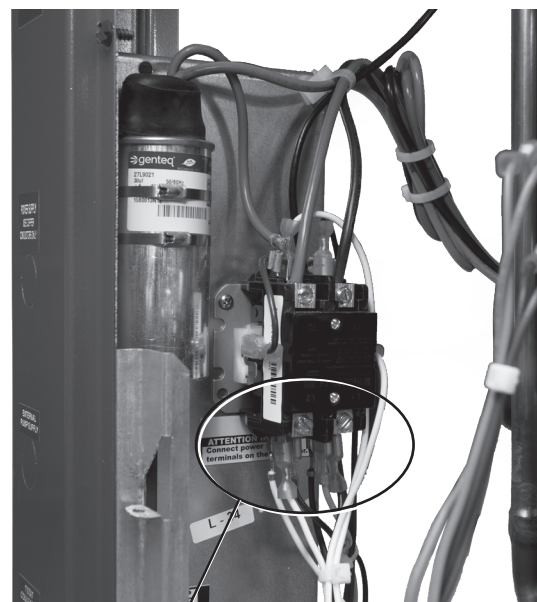
Figure 24: Tranquility® Single Phase Line Voltage Field Wiring
