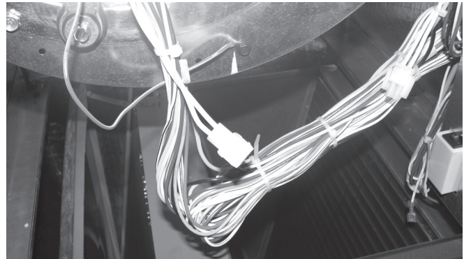
Figure 11: Remove Harness Plug
