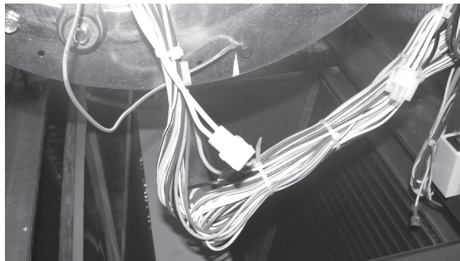
Figure 9: Install 2-Pin Jumper Plug
