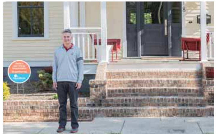
Geothermal can be installed almost anywhere, even in small lots. For Harrell's home, boreholes for the geothermal loop were drilled on both sides of the porch.
