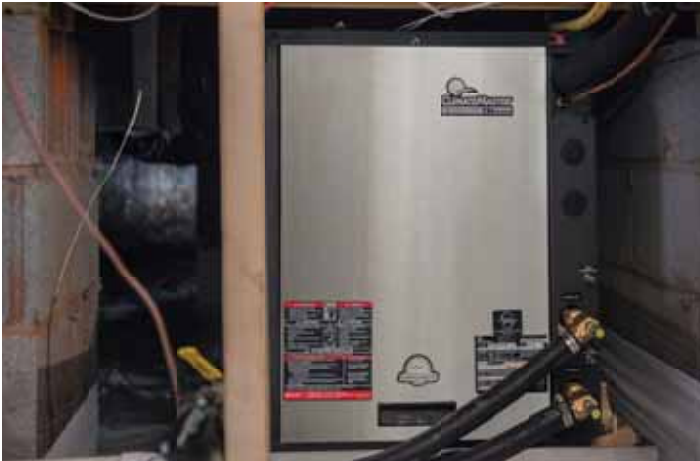
One of two units in Harrell's home, this is the Tranquility® Digital Indoor Split (TES) Geothermal Heat Pump. The TES can be installed in an attic, basement or crawl space.
