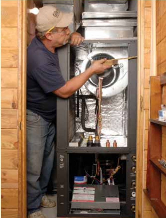
An F.W. Behler contractor installs a ClimateMaster TTV unit.
