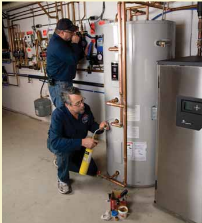
F.W. Behler contractors finishing up the THW installation.
