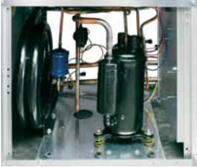
Double spring and grommet compressor isolation
