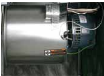
Torsion-flex blower motors
