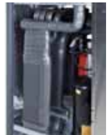
Fully Insulated Water and Refrigerant Lines
