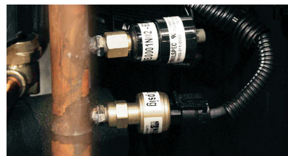
Figure 41 - Discharge Pressure Transducer
