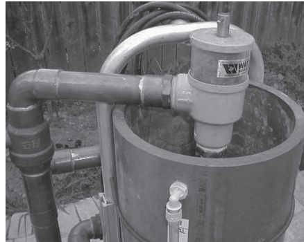
Figure 8b: Cam Fittings for Flush Cart Hoses
